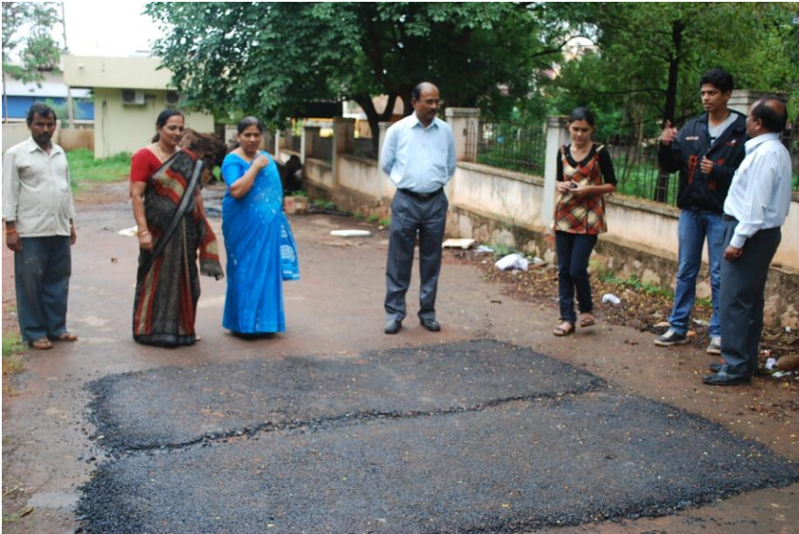
Principle and HOD observing the completed road
